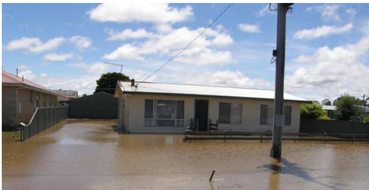
A Miners Rest house flooded above floor during the January 2011 flood event (source: City of Ballarat).
