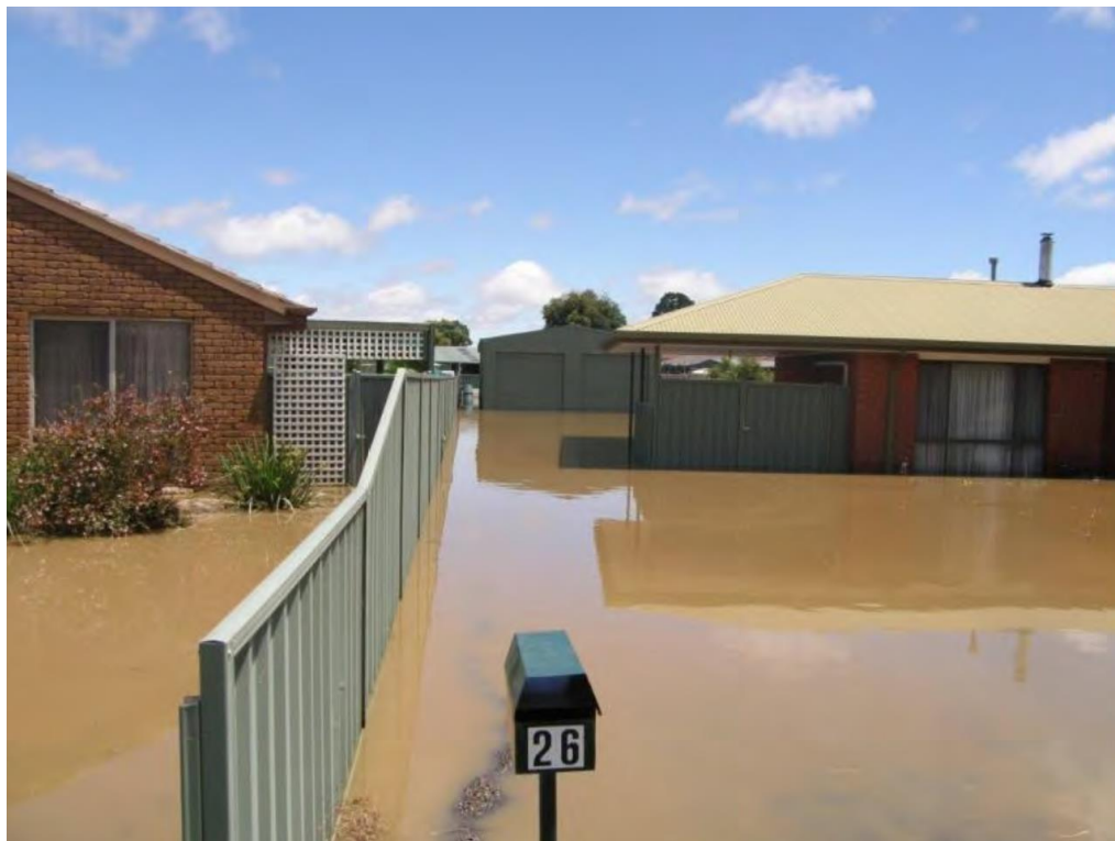
A Dundas Street house flooded above floor in Miners Rest during the January 2011 flood event (source: City of Ballarat).
