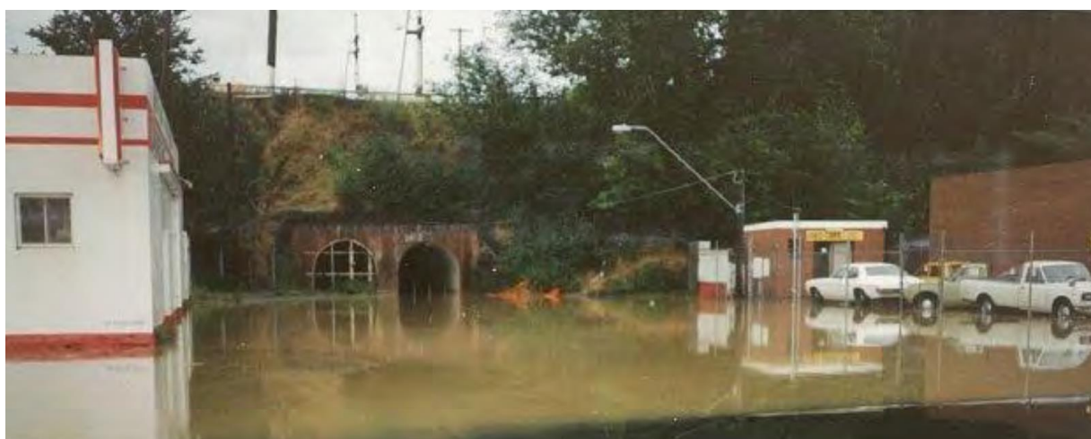
Flooding along Davies Street pedestrian culverts from Yarrowee River during the 1991 flood event (City of Ballarat 2016).
