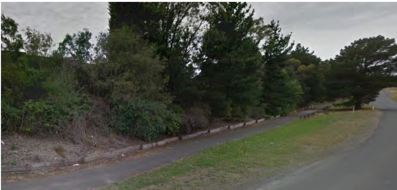
Charlesworth Street embankment.
