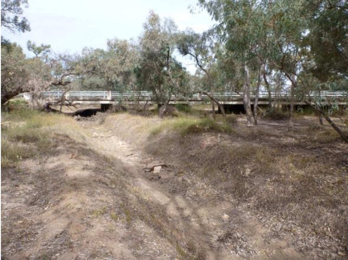
Fig A3-1. Calder Hwy Bridge
