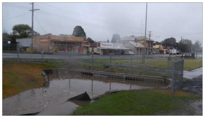
Figure 4. New culverts in Montgomery Street, during the September 2016 flood event.
