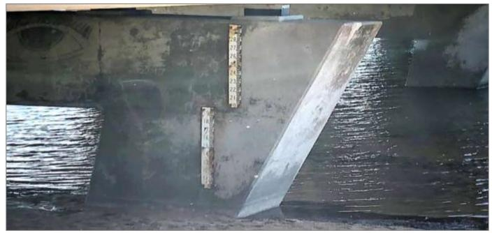
Figure 60. Curdies Inlet gauge board on the Peterborough Bridge.
