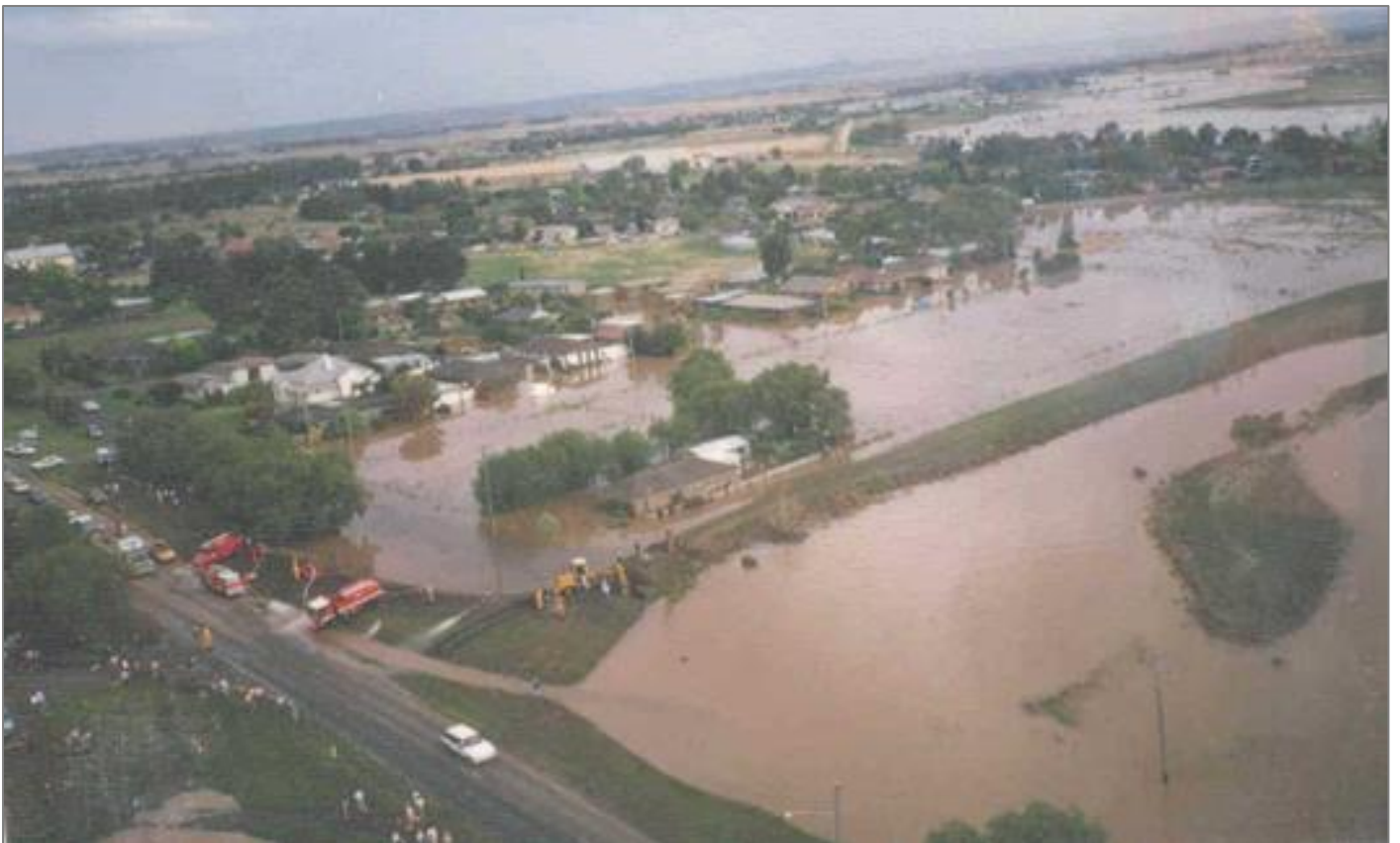
Figure 23. Flooding impacting Station Lake Road, Lara during the 1988 event (Water Technology 2019).
