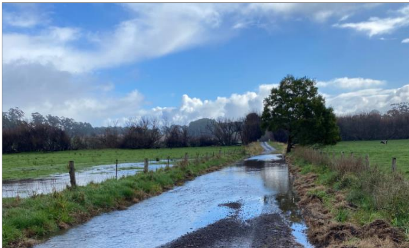
Figure 13. Deep flooding caused by the West Barwon Reservoir spill in July 2021, cutting access to Boundary Road, along the Barwon River West Branch.
