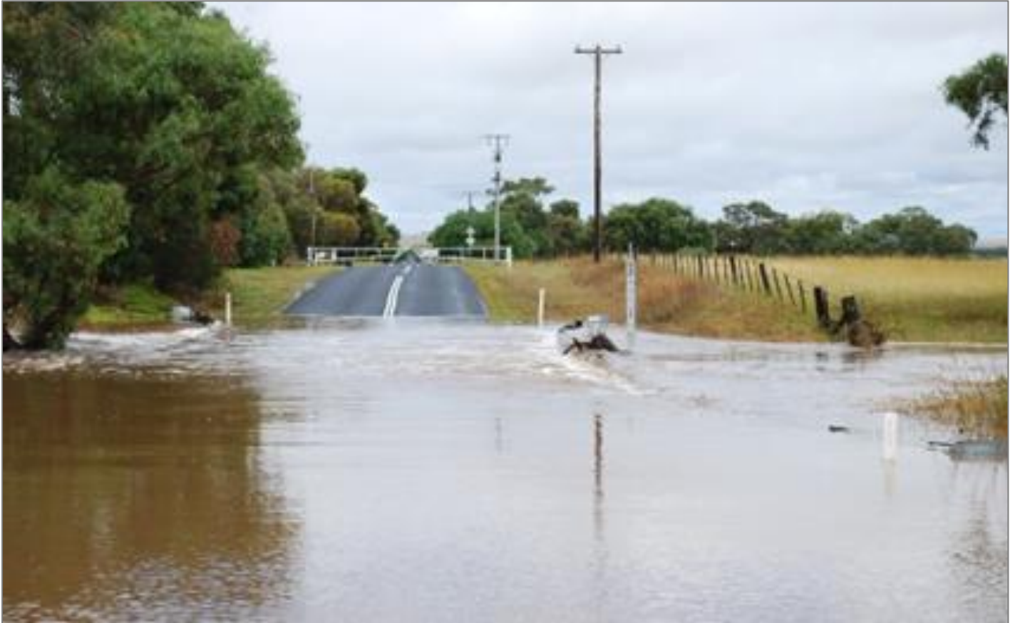
Figure 25. Deep flooding along Windermere Road during the January 2011 event (Water Technology 2019).
