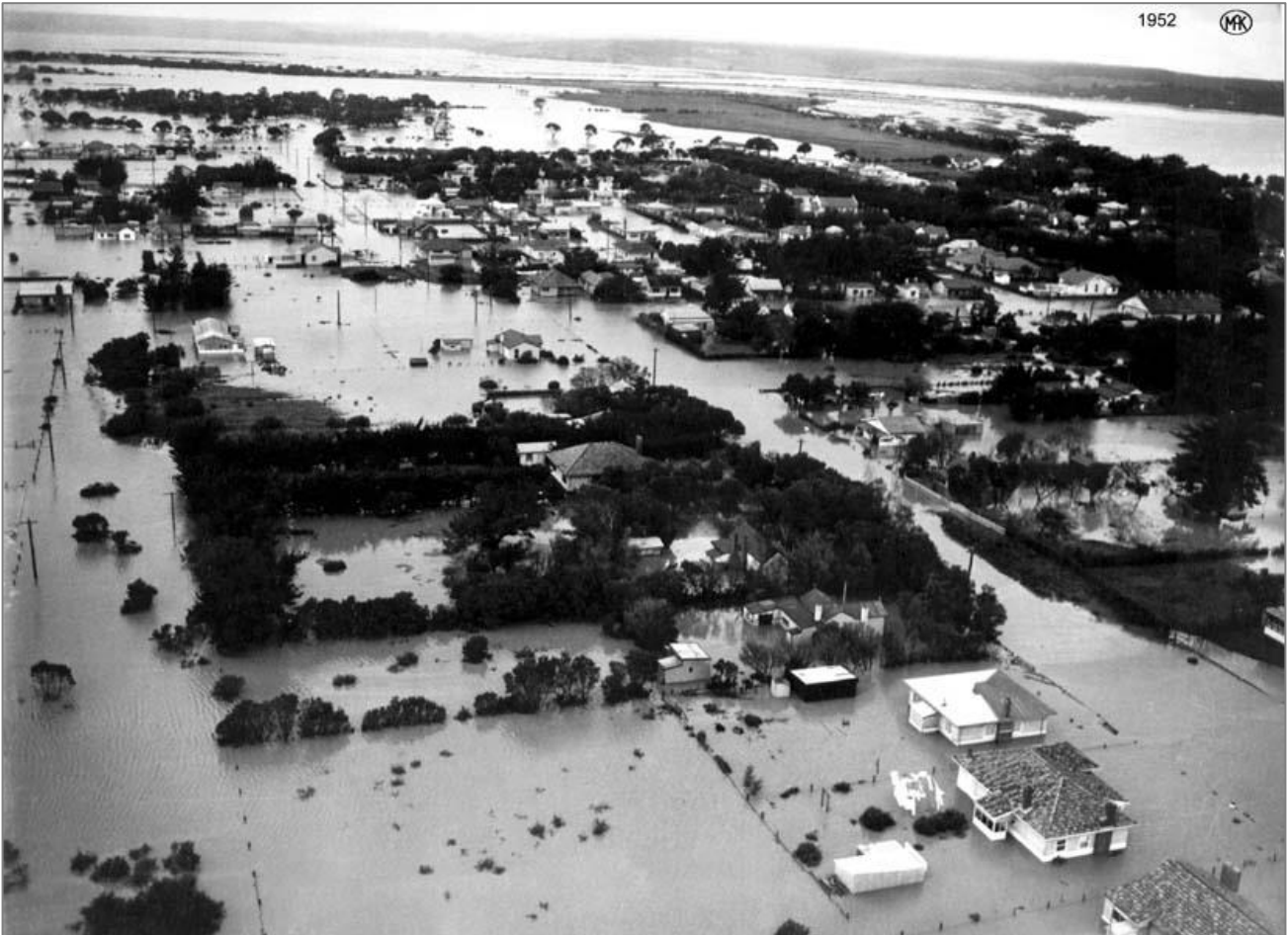
Figure 91. Flooding impacting Barwon Heads during the 1952 event (Barwon Heads Heritage Association).
