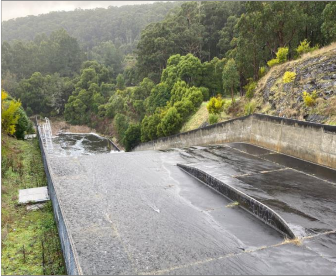
Figure 12. West Barwon Reservoir spillway, July 2021.
