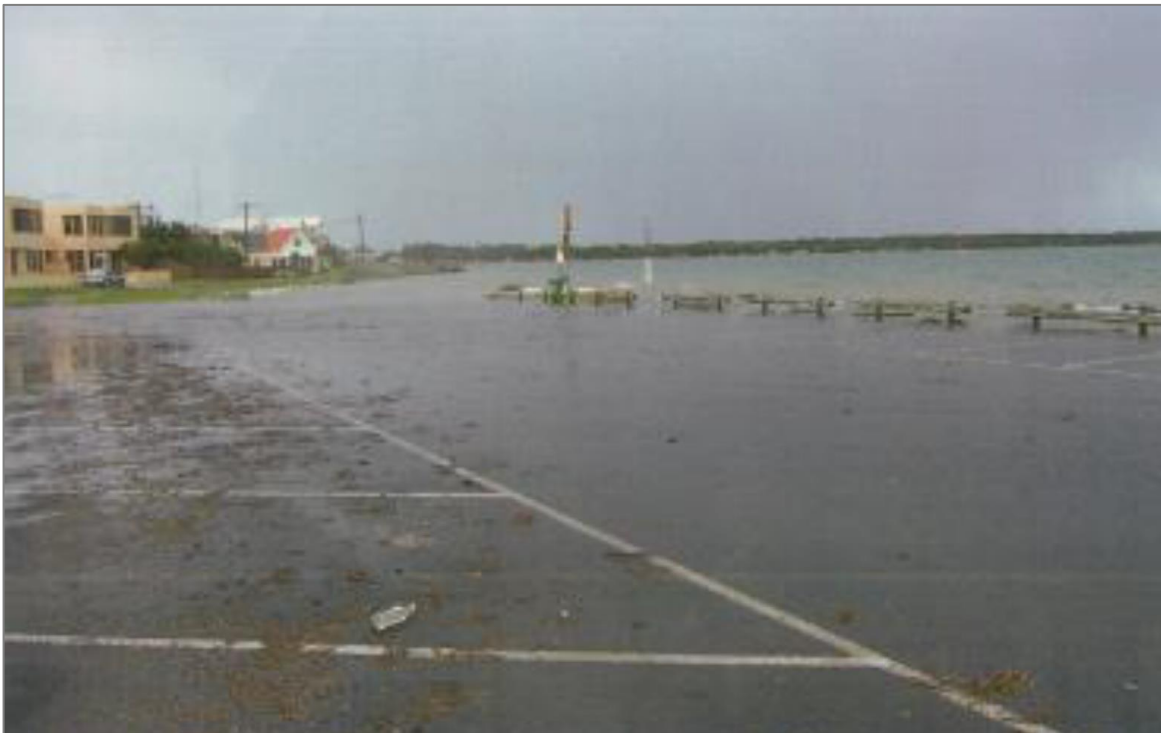
Figure 96. Flooding impacting the Ocean Grove Boat Ramp during the 2004 event (COGG 2018).
