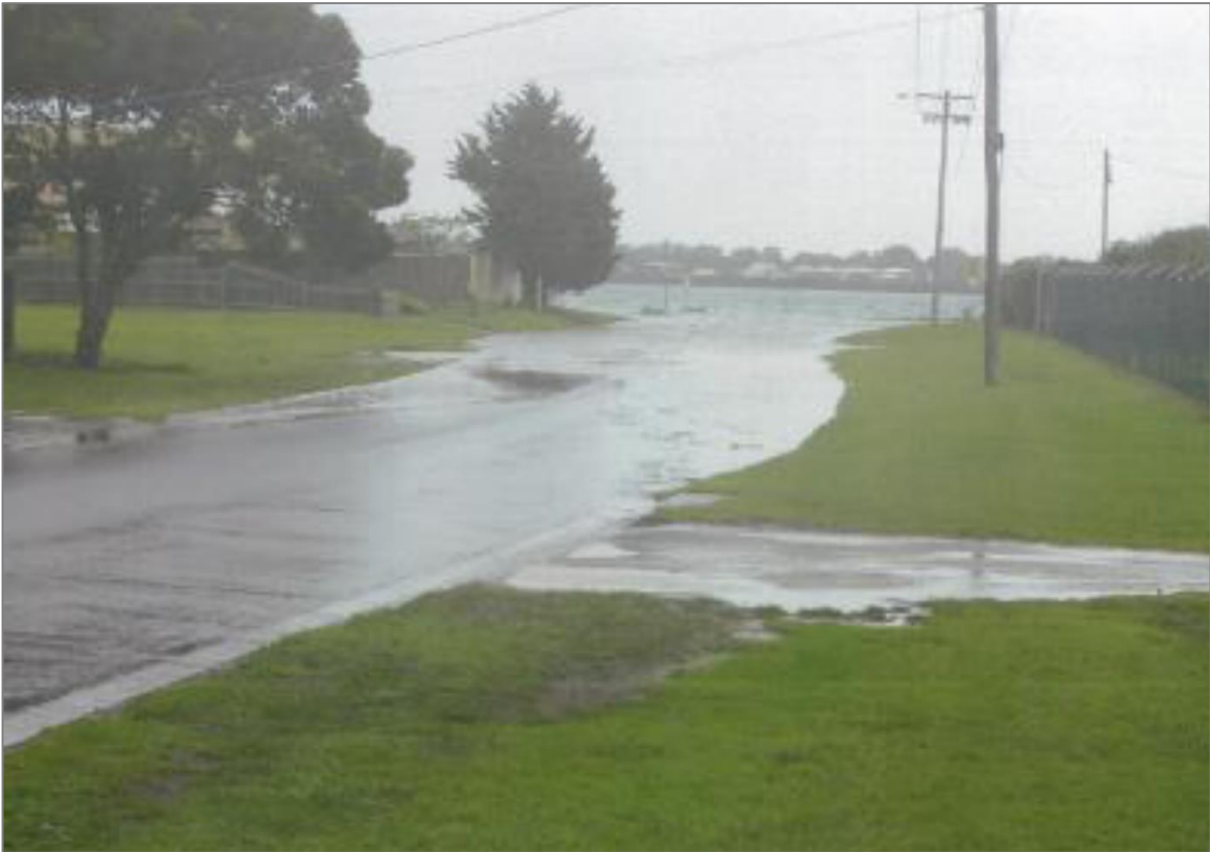
Figure 97. Flooding impacting Guthridge Street, Ocean Grove during the 2004 event (COGG 2018).
