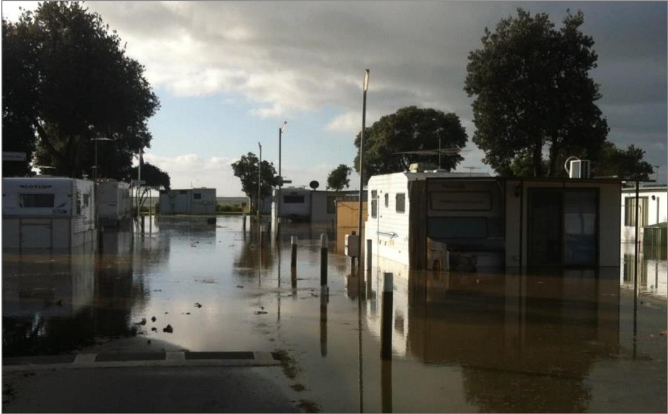
Figure 3. Storm surge flooding at the Portarlington Caravan Park during the June 2014 storm surge flood event (COGG 2018).
