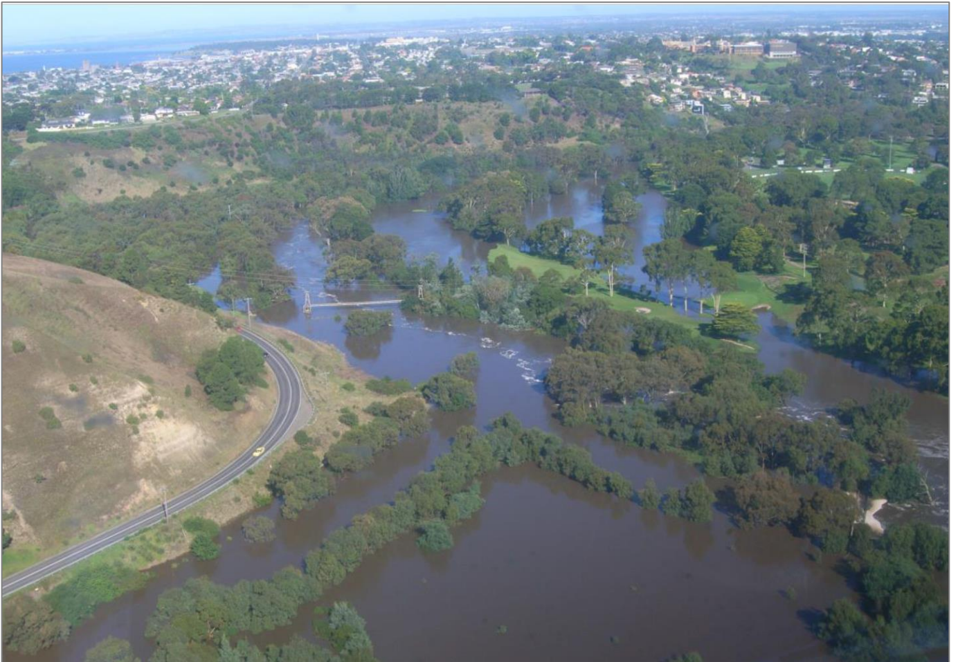
Figure 65. Flooding along Queens Park, Geelong during the January 2011 flood event (Water Technology 2016).
