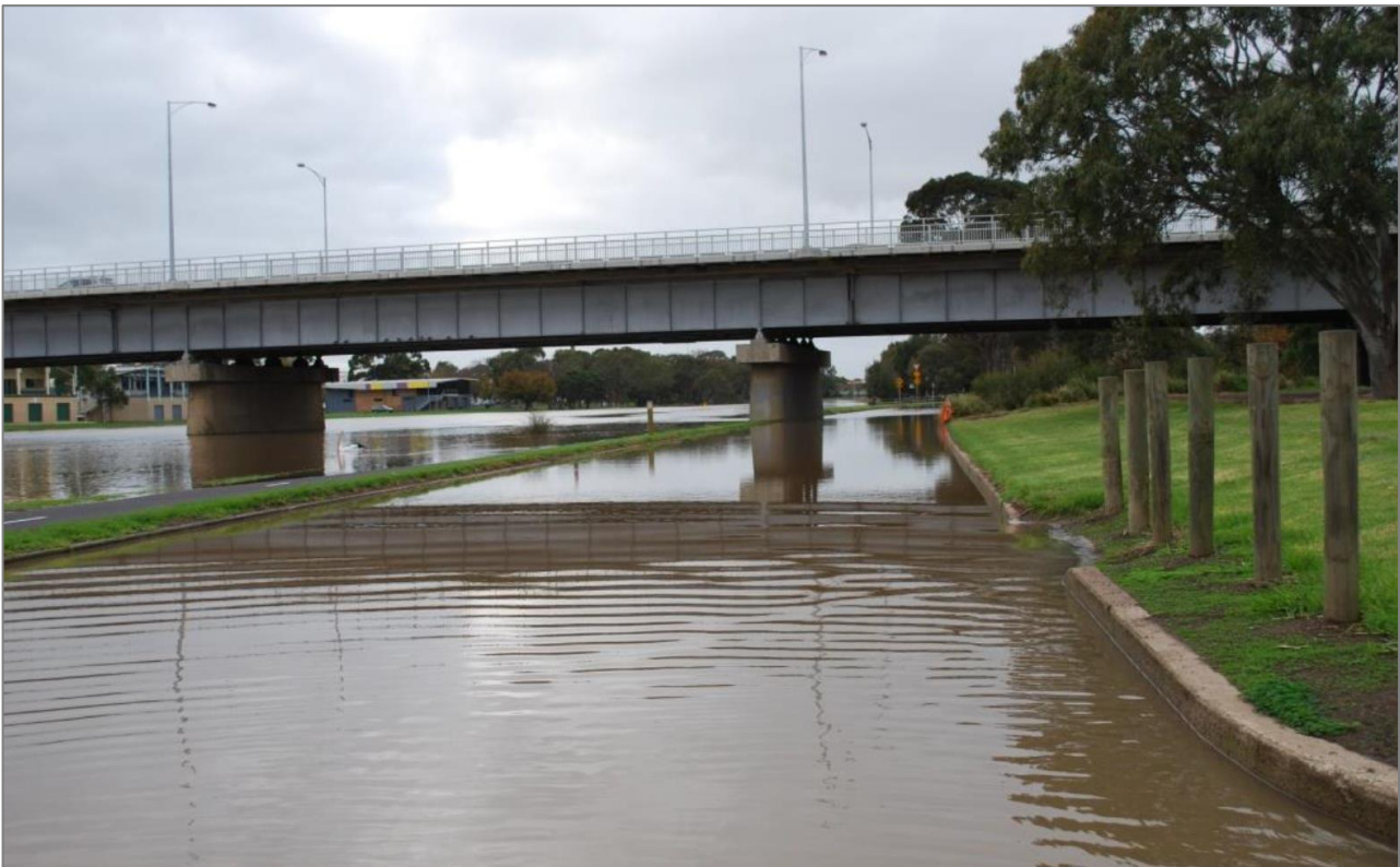
Figure 68. Flooding adjacent to Geelong Rowing Clubs and the Moorabool Street Bridge during the January 2011 flood event (COGG 2018).
