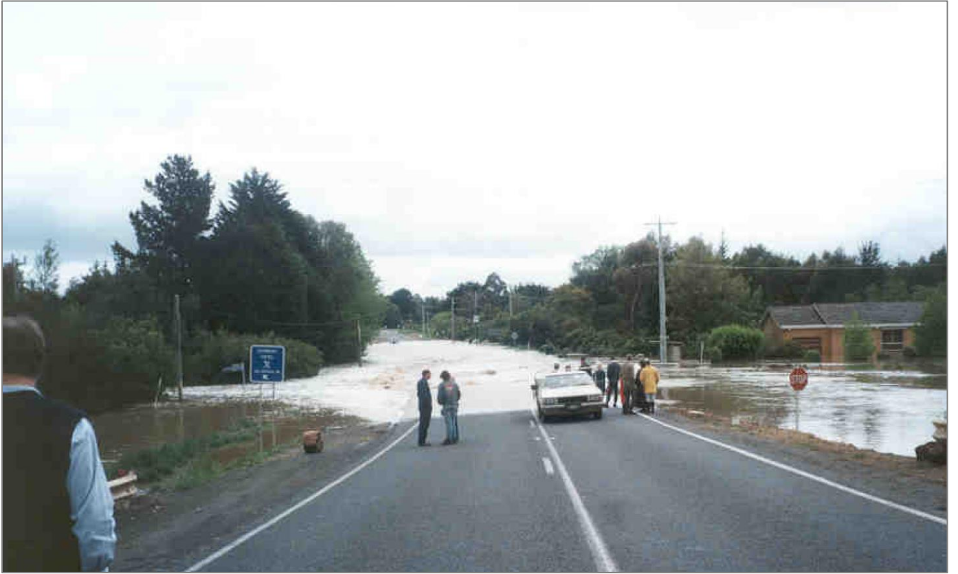
Figure 53. Flooding adjacent to the Midland Highway Bridge during the 1995 flood event.
