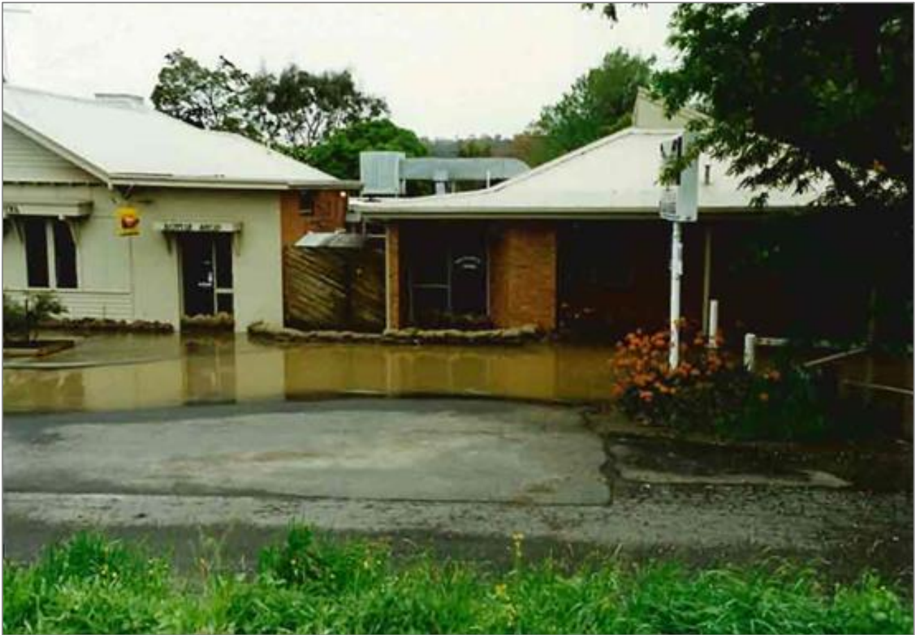
Figure 51. Flooding at the Batesford Hotel during the 1995 flood event.
