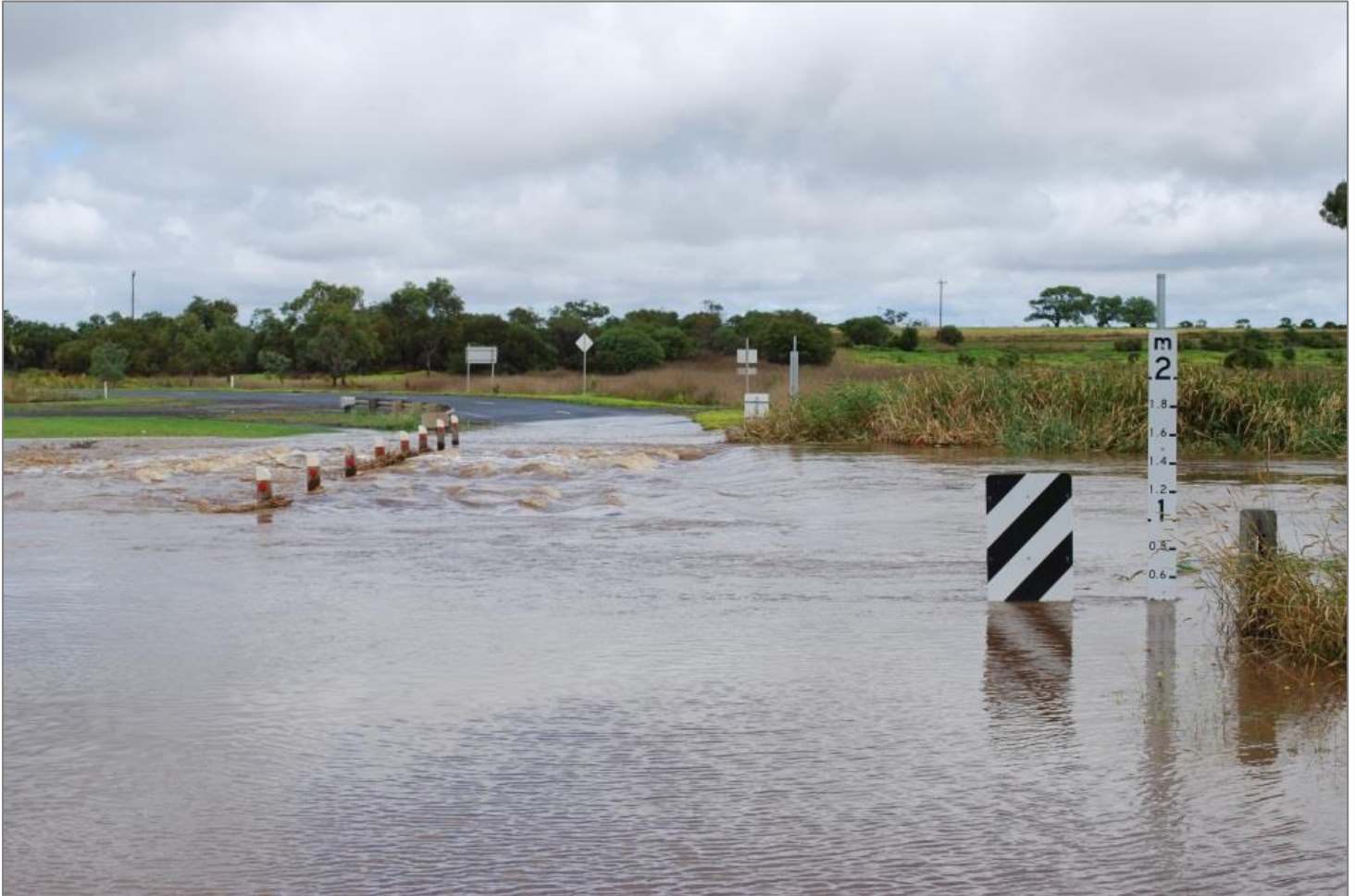
Figure 22. Flooding impacting the Rennie Street floodway during the 2011 flood event (Water Technology 2019).
