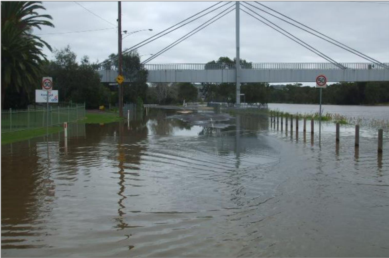
Figure 67. Flooding looking west along Barrabool Road, Geelong during the January 2011 flood event (COGG 2018).
