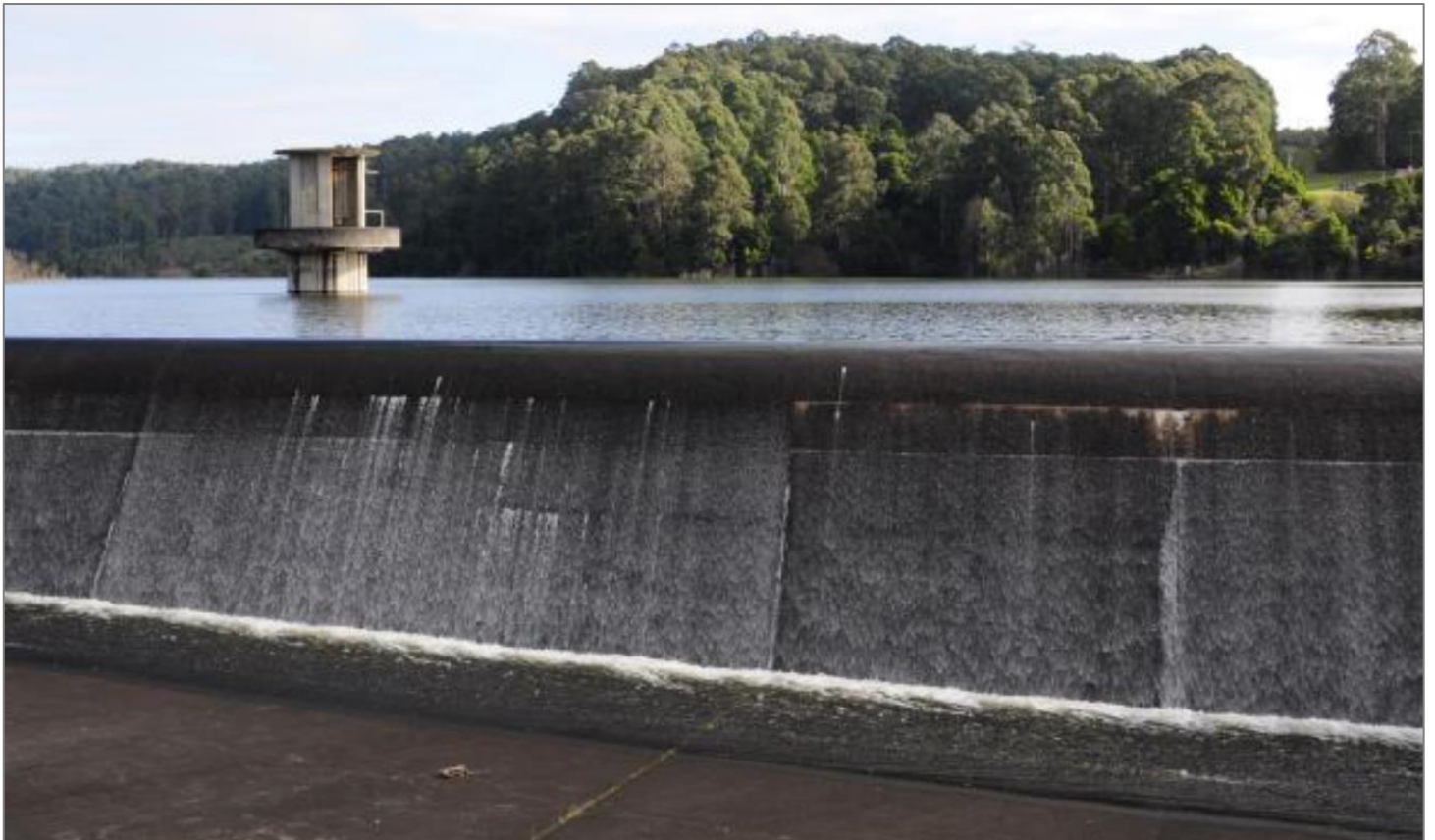
Figure 11. West Barwon Reservoir spillway.
