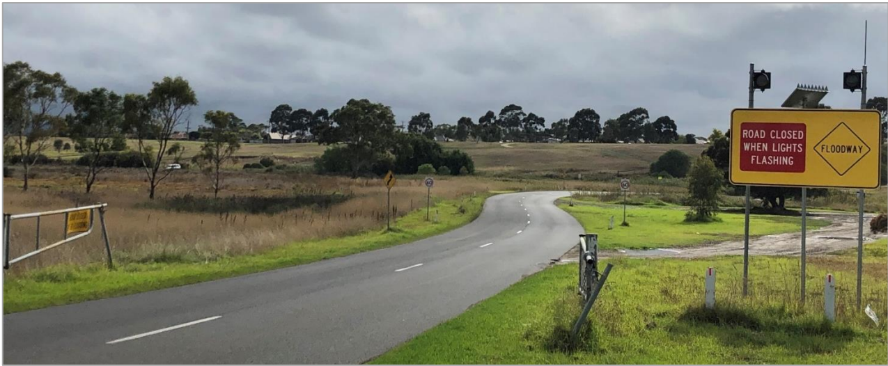
Figure 18. Rennie flood gate and flood warning signs at the Hovells Creek floodway south of Lara, adjacent to the Princes Freeway.
