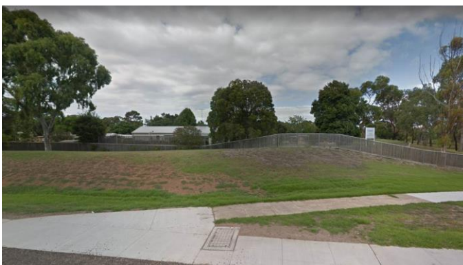
Lara Levee at Station Lake Road
