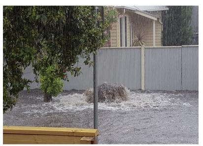
This occurs because drains are designed to transport a limited capacity of water. See an example of this to the left.
