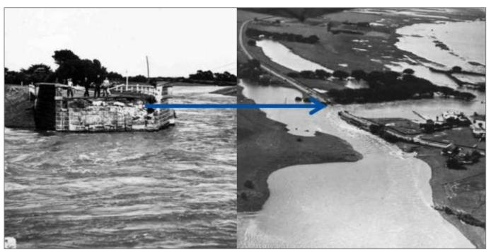
Figure 7. The Rosebrook Bridge along the Princes Highway washed away in the 1946 flood.
