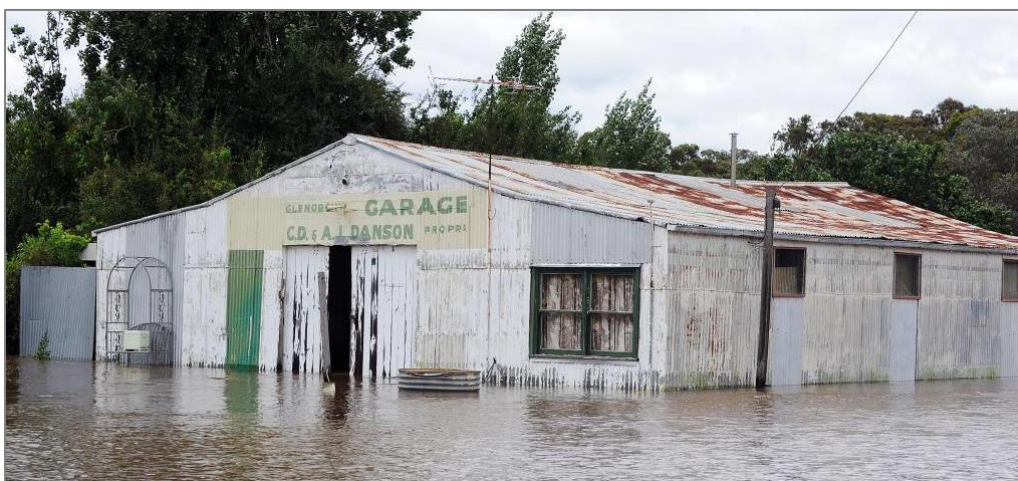
Flooding impacting a Garage in Forest Street, Glenorchy during January 2011 .
