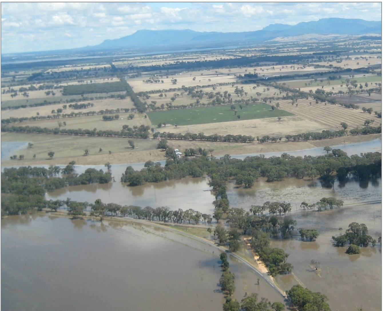
Flooding overtopping the Stawell-Warracknabeal Road, north-west of Glenorchy during January 2011.
