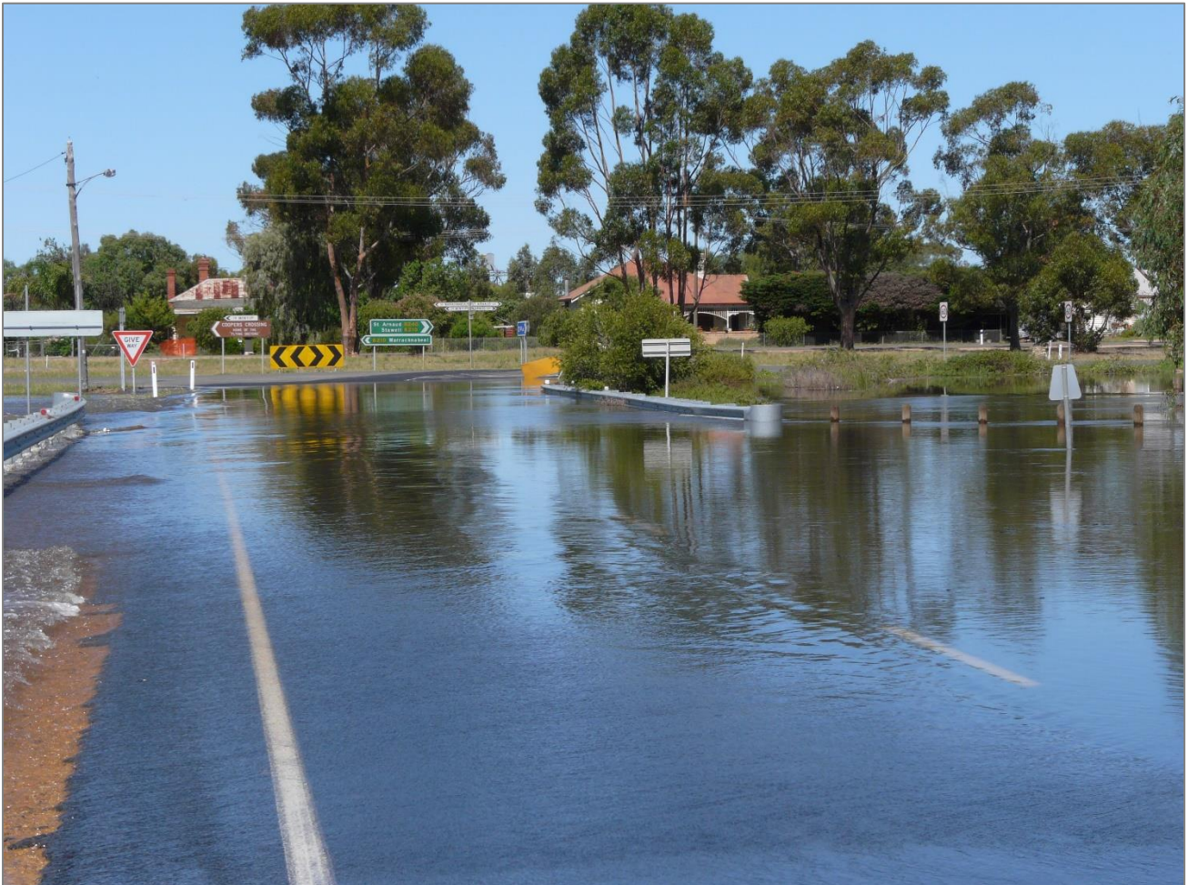
Flooding overtopping the Wimmera Highway north of Rupanyup during January 2011.
