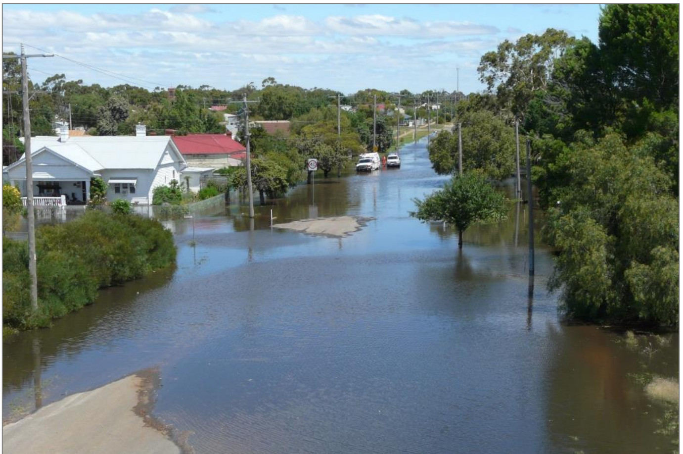
Flooding impacting Dyer Street, Rupanyup during January 2011 event.
