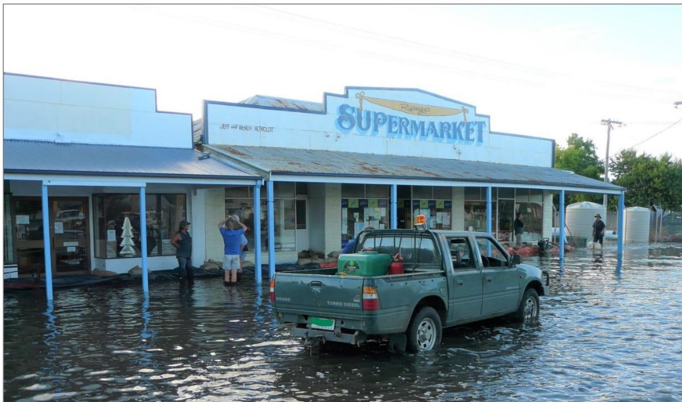
Flooding impacting the old Rupanyup Supermarket during January 2011 event.
